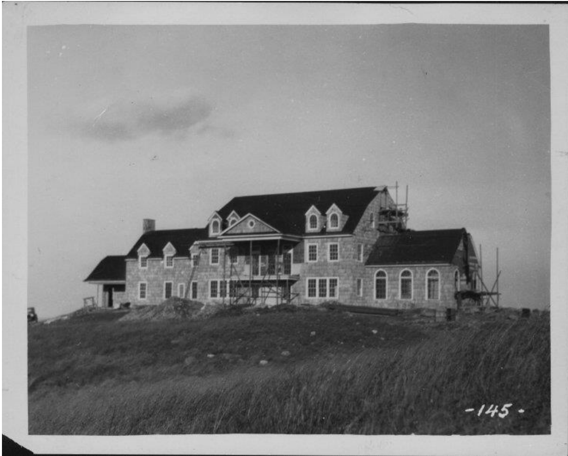
Photograph of the Carl Fisher House under construction, Judy Sauers Collection, Montauk Library Archives.
